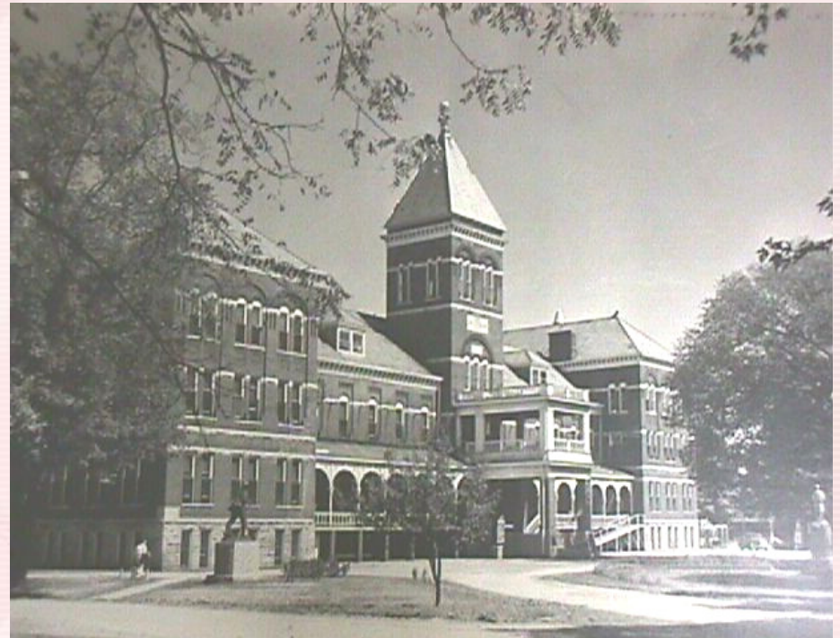
The Main Building (capacity 200 residents)
